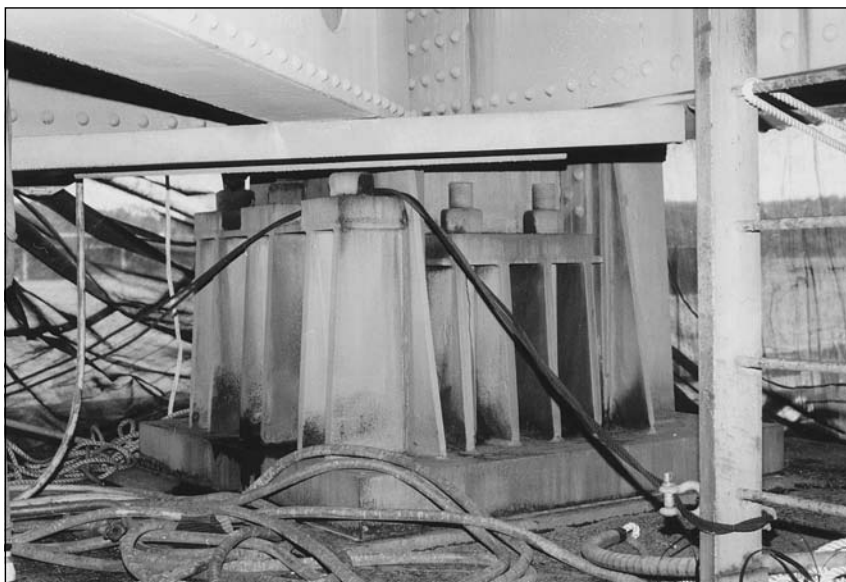
Figure 4.19 Some bearings, like the one shown above, can be quite massive in size.
