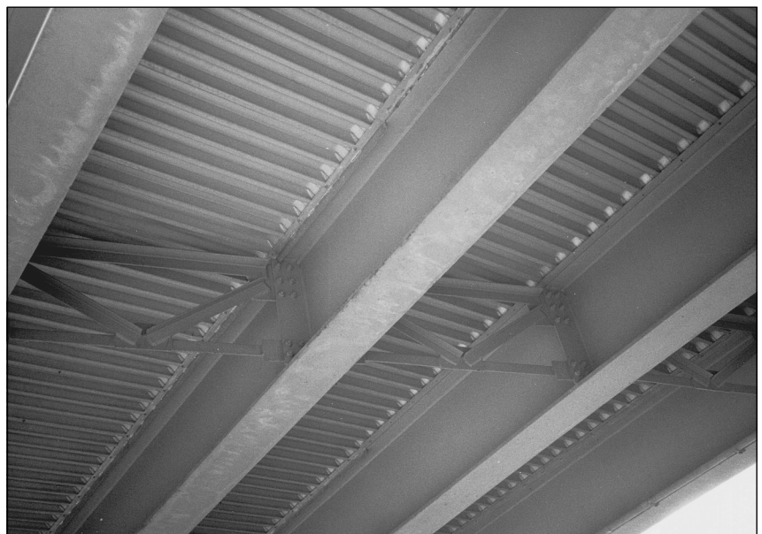
Figure 2.8 Stay-in-place forms can hide deterioration beneath them.
