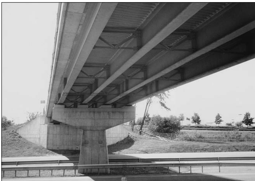
Figure 1.5 A hammerhead pier supports a slab-on-stringer superstructure.
