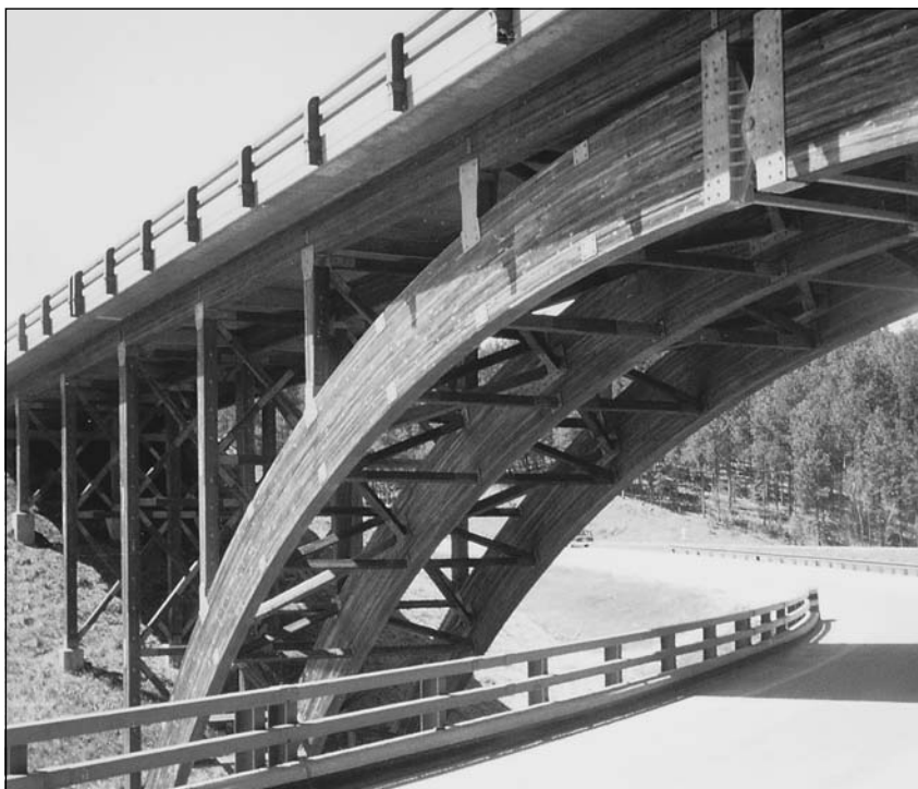
Figure 3.4 Timber was used to construct this open spandrel arch bridge in South Dakota.
