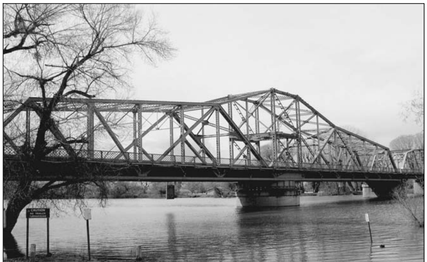
Figure 1.14 American River Bridge near Sacramento, California.
