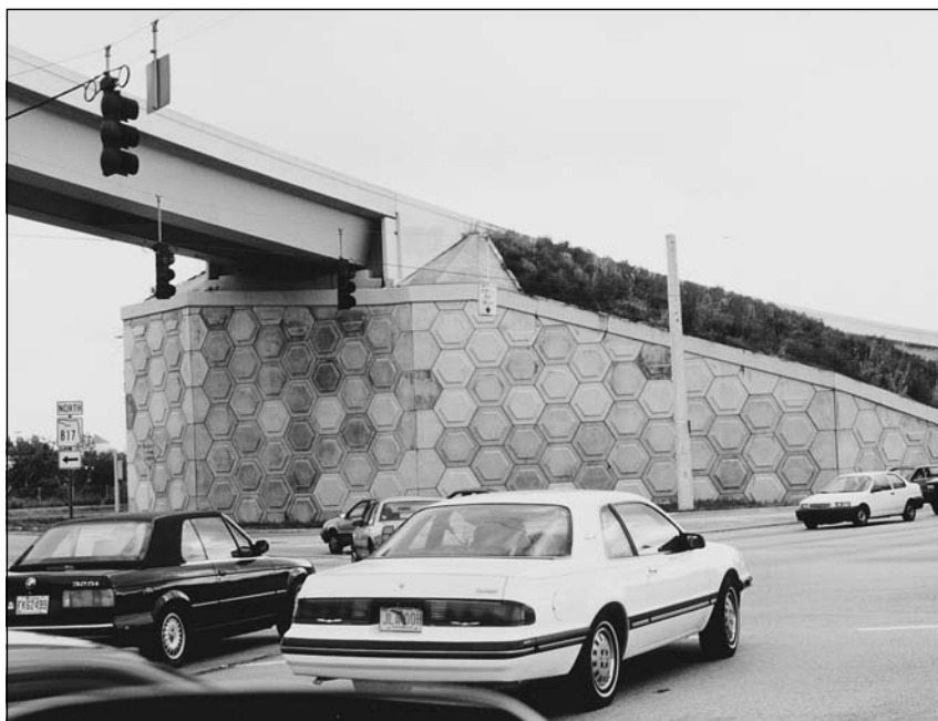
Figure 4.2 A reinforced earth abutment is used to support this composite steel bridge.
