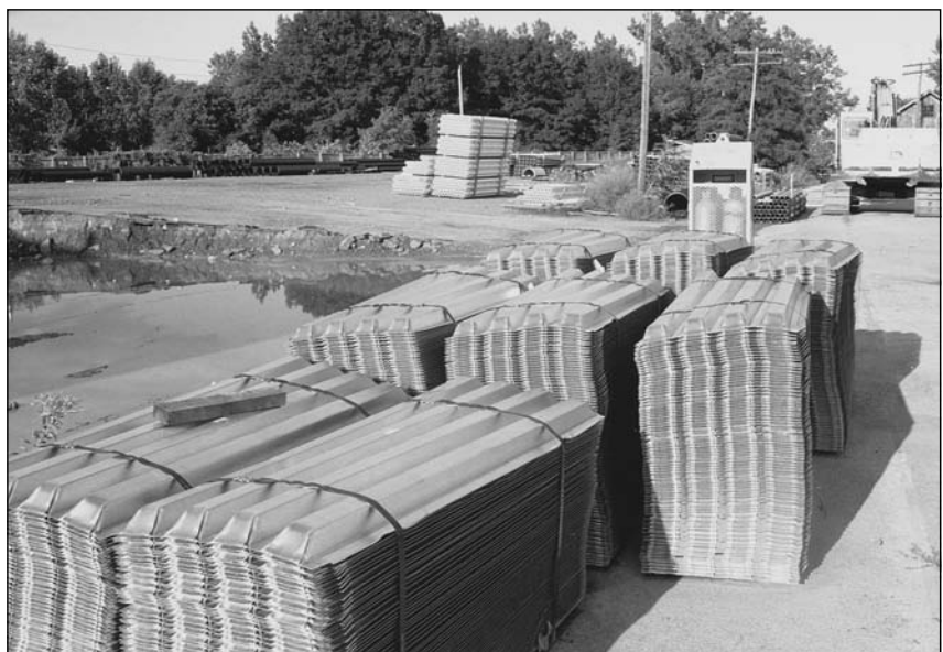
Figure 3.34 Steel deck forms, like those above, can affect composite construction.
