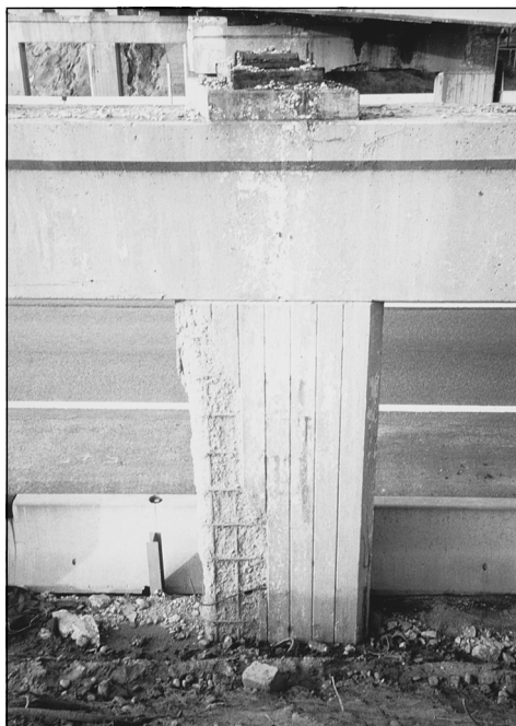
Figure 2.6 Exposed reinforcing signals repair.
