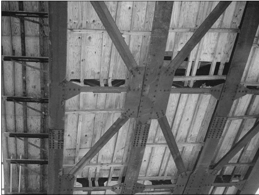
Figure 1.4 Lateral bracing on a horizontally curved steel girder bridge.
