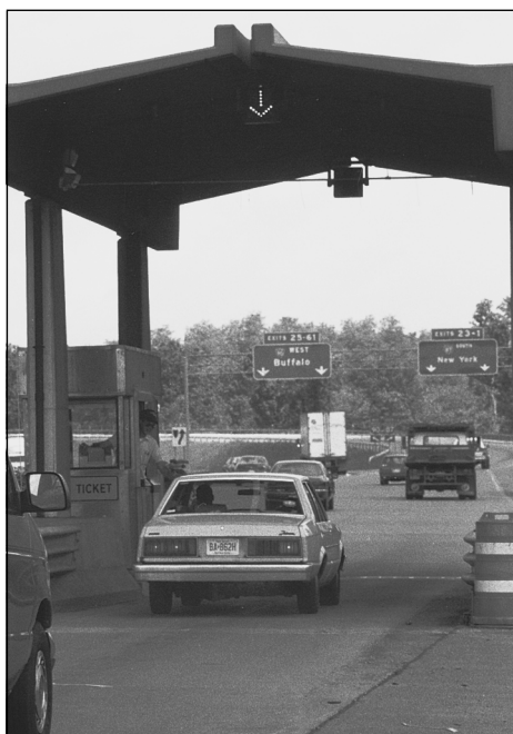
Figure 2.1 Toll roads, such as the NYS Thruway, are principally found in the northeastern U.S.
