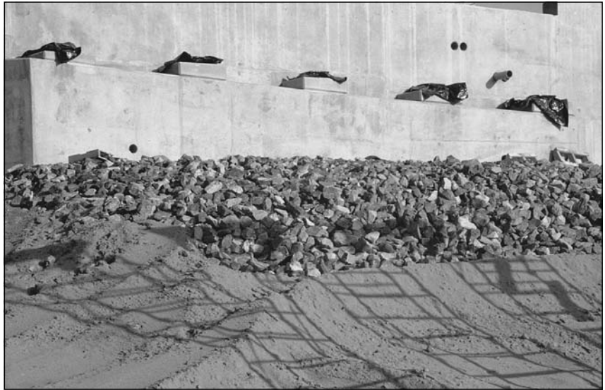
Figure 1.9 Broken rocks, varying in size, can be used as slope protection.
