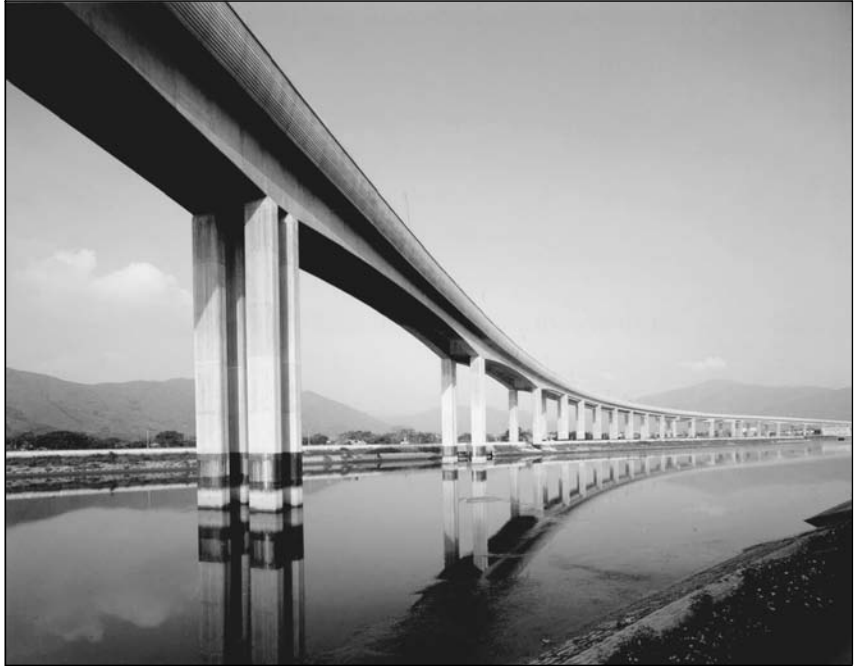
Figure 1.11 KCRC West Rail Viaducts, Hong Kong.
