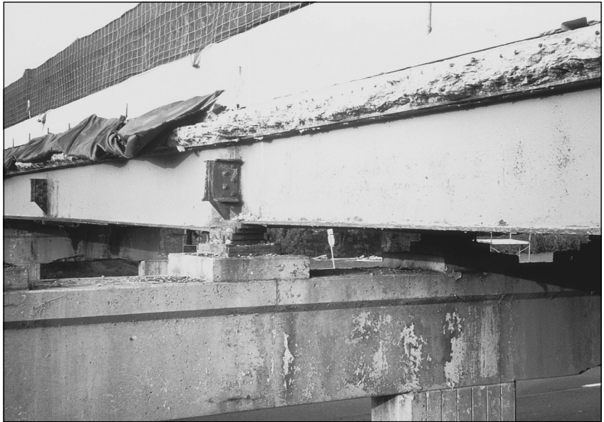
Figure 2.3 There is plenty room for improvement in the way bridges are designed.
