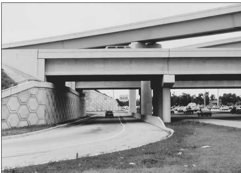
Figure 3.54 A steel plate girder structure passes over a prestressed concrete bridge in Florida. Steel and prestressed concrete often coexist in the same environment.
