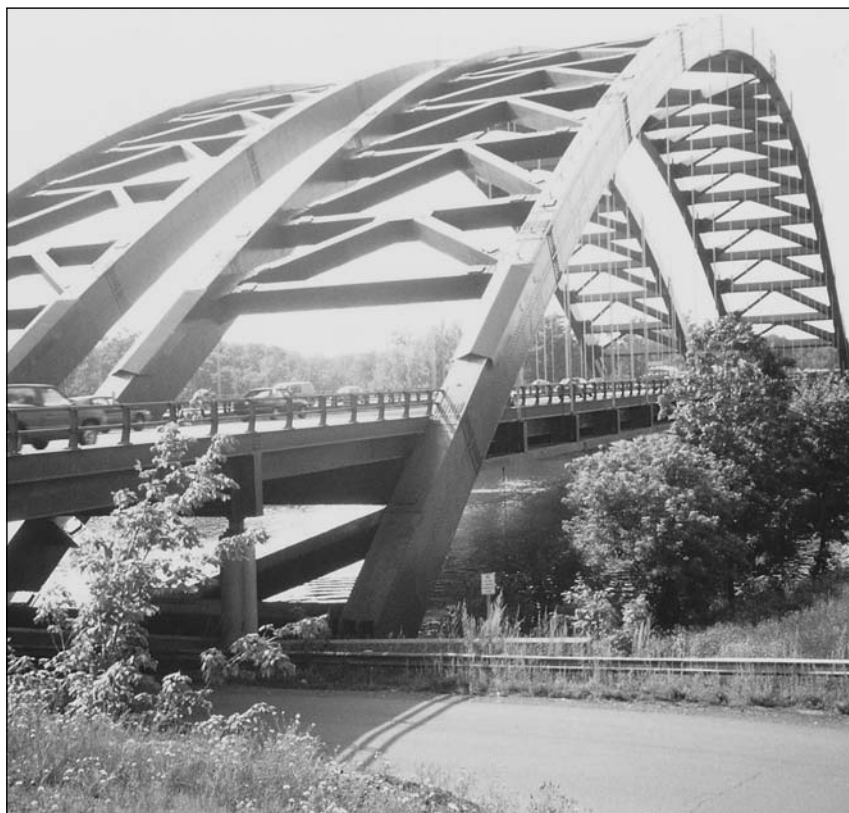
Figure 1.13 Twin steel through arches cross the Mohawk River in upstate New York.
