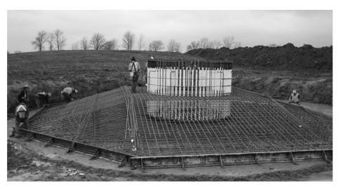
Fig. 1-2 Wind turbine foundation. (Photograph courtesy of Invenergy.)
