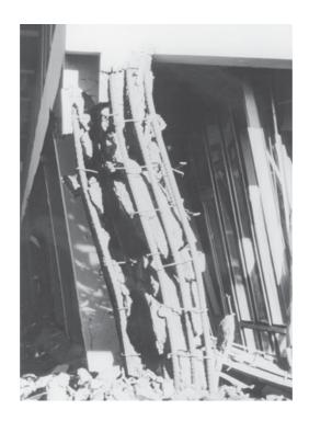
Fig. 11-6 Tied column destroyed in 1971 San Fernando earthquake. (Photograph courtesy of National Bureau of Standards.)
