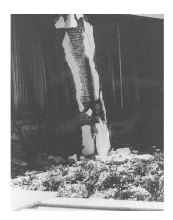
Fig. 11-7 Spiral column damaged by 1971 San Fernando earthquake. Although this column has been deflected sideways 20 in., it is still carrying load. (Photograph courtesy of National Bureau of Standards.)
