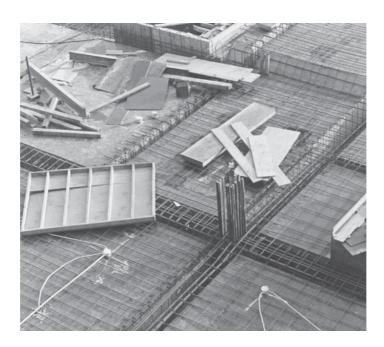
Fig. 5-22 Intersection of a column and two beams.
